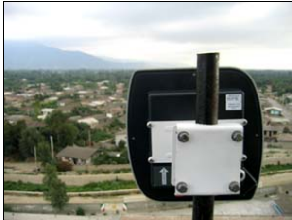
Residents in three villages can now access government services through the wireless network
